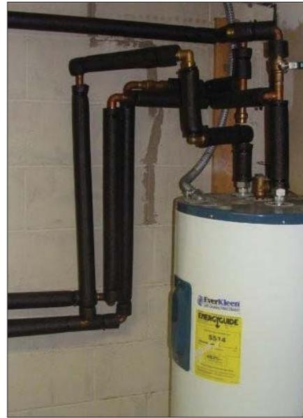
**Above: Clark's water heater piped to the geothermal system. Bottom Left: Refrigeration pumps that produce the heat. Photos by Louis & Wanda Clark.**
