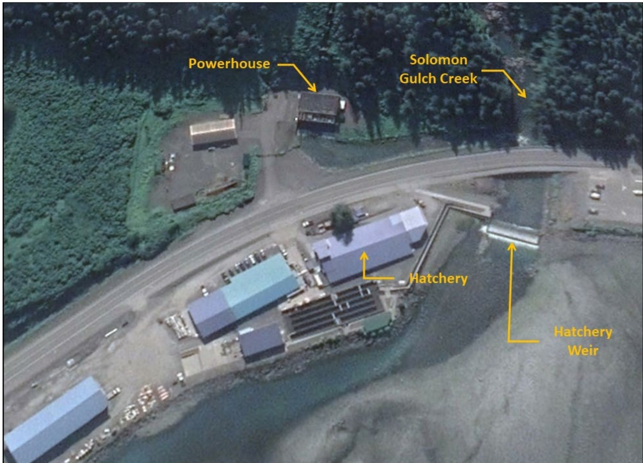
Photo 3-1 Solomon Gulch Hydroelectric Powerhouse and Tailrace, VFDA Hatchery, and the Mouth of Solomon Gulch Creek
