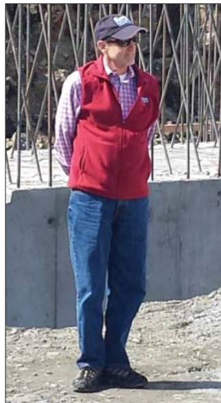
CEO Wilkinson looks on from in front of the foundation of the Powerhouse
