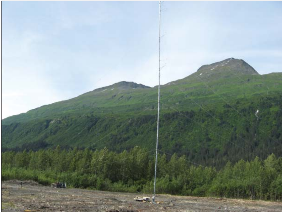
The CVEA MET tower is located in the center of a clearing 200 feet in radius. It stands 167 feet in the air and is supported by 12 anchors and 20 guy wires.
