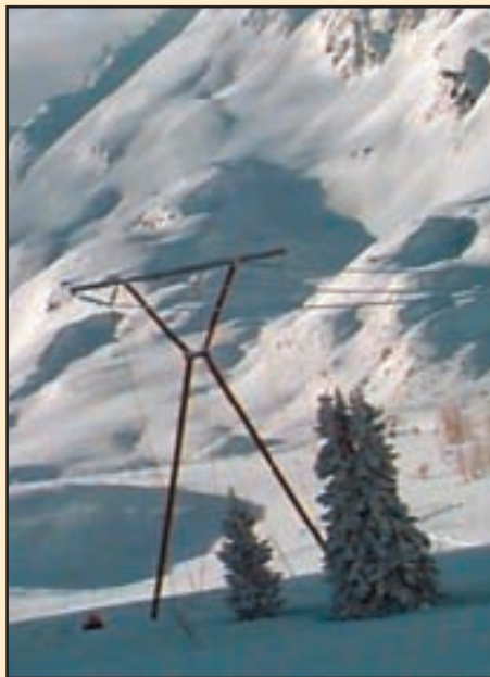
The Four Dam Pool transmission line, Thompson Pass, Alaska.
