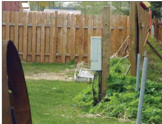
Above, two CVEA rights of way (ROW); the left has many objects in the ROW and might impede quick response if access is needed, the one on the right has been cleared as part of the ROW maintenance program
