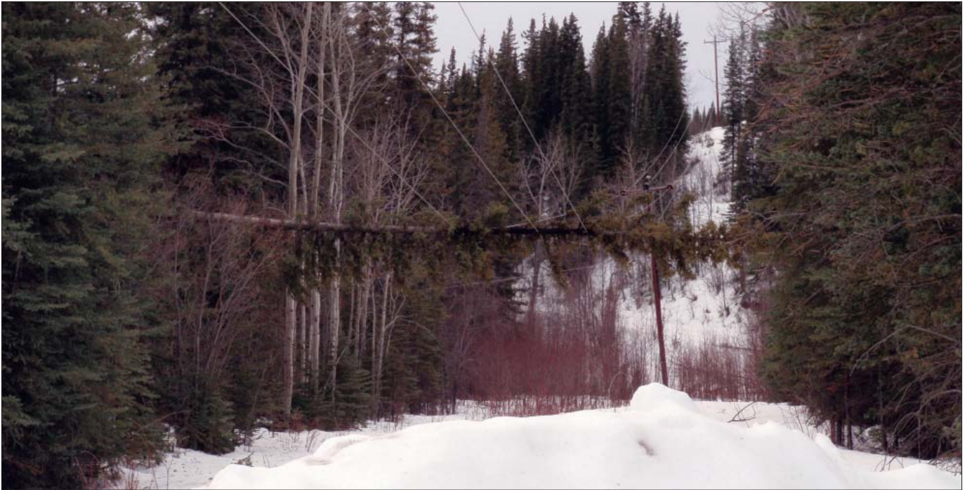
Above, a tall tree from far outside CVEA's right of way in the Copper Basin fell into the power line Opposite left, multiple trees from outside CVEA's right of way were forced into power lines by heavy, wet snow during a severe weather storm in the Copper Basin Opposite right, a tree on the power line due to heavy wind caused a widespread outage
