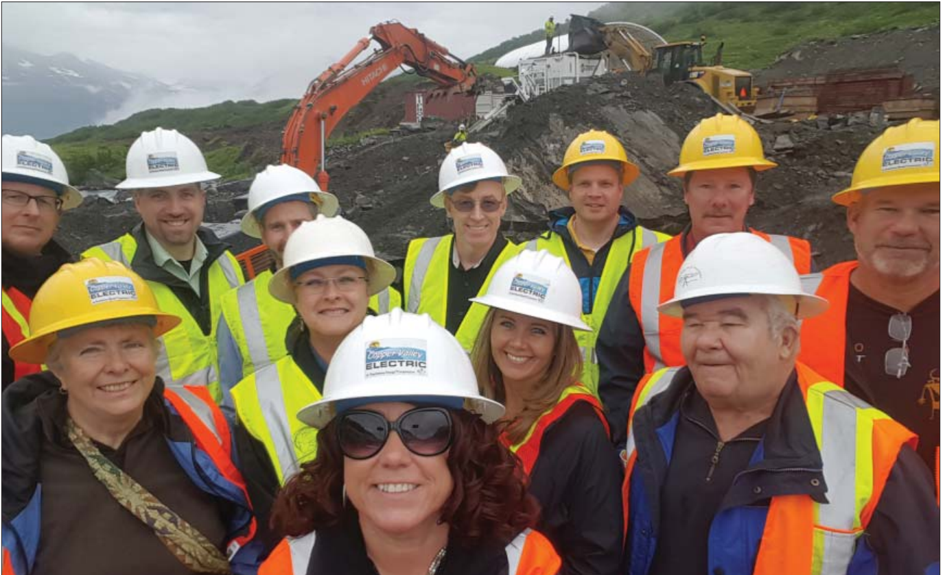
The CVEA Board of Directors joined Co-op Staff on a tour of the Allison Creek Hydroelectric Project construction site in 2015 Photo by Sharon Crisp
