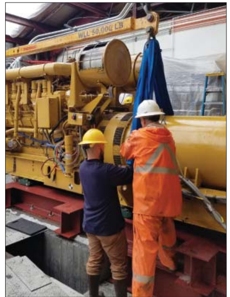
Opposite, Valdez Plant Operator Ryan Compehos and Valdez Line Foreman Todd Stahley prepping one of the replacement gensets to be lifted and set in the VDP by crane
