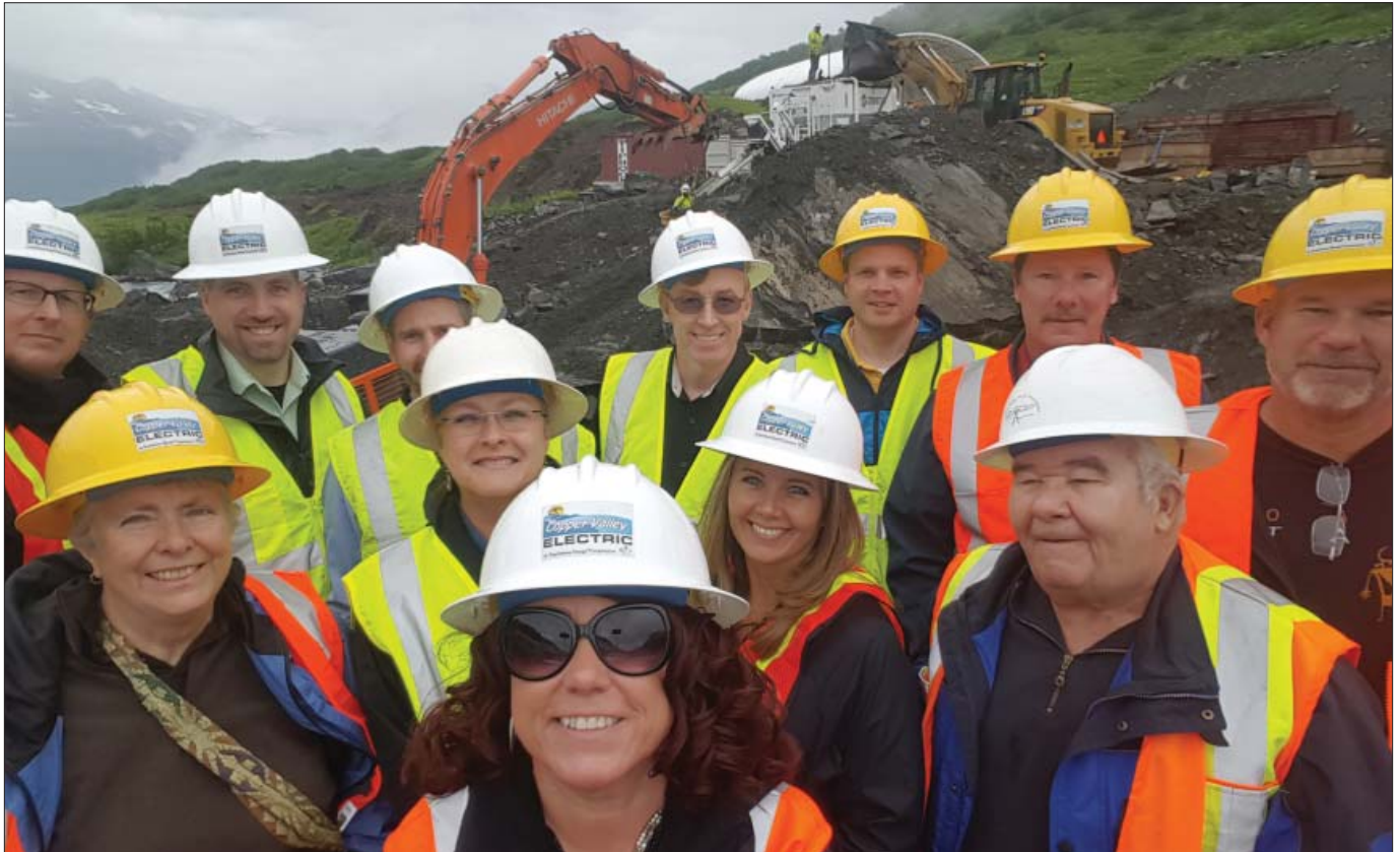
The CVEA Board of Directors joined Co-op Staff on a tour of the Allison Creek Hydroelectric Project construction site in 2015 Photo by Sharon Crisp
