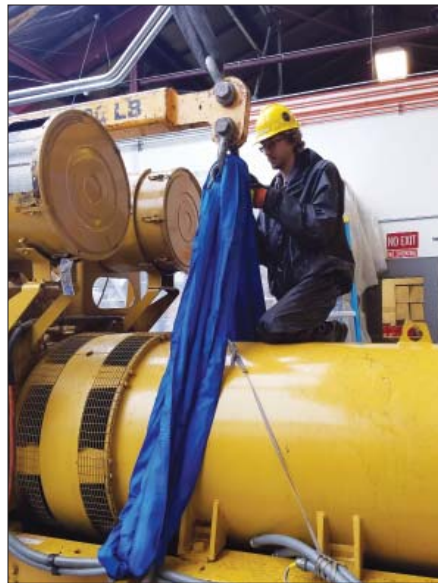
Opposite, Valdez Plant Operator Ryan Compehos and Valdez Line Foreman Todd Stahley prepping one of the replacement gensets to be lifted and set in the VDP by crane
