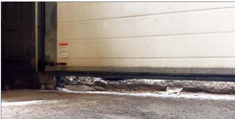
Top Left, the site of the new building on the CVEA grounds Above, dirt work on the site, preparing for low grade electrical and plumbing installation Left, garage door of current building; the door cannot close due to foundation shifting leaving a roughly six inch gap
