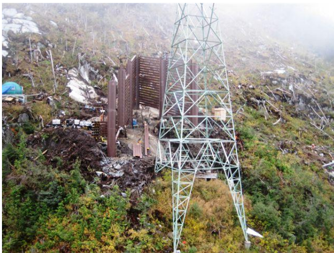
Snettisham Splitting Wedge Structure
