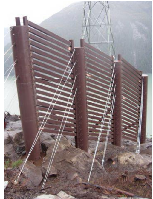
Snettisham Splitting Wedge Structure
