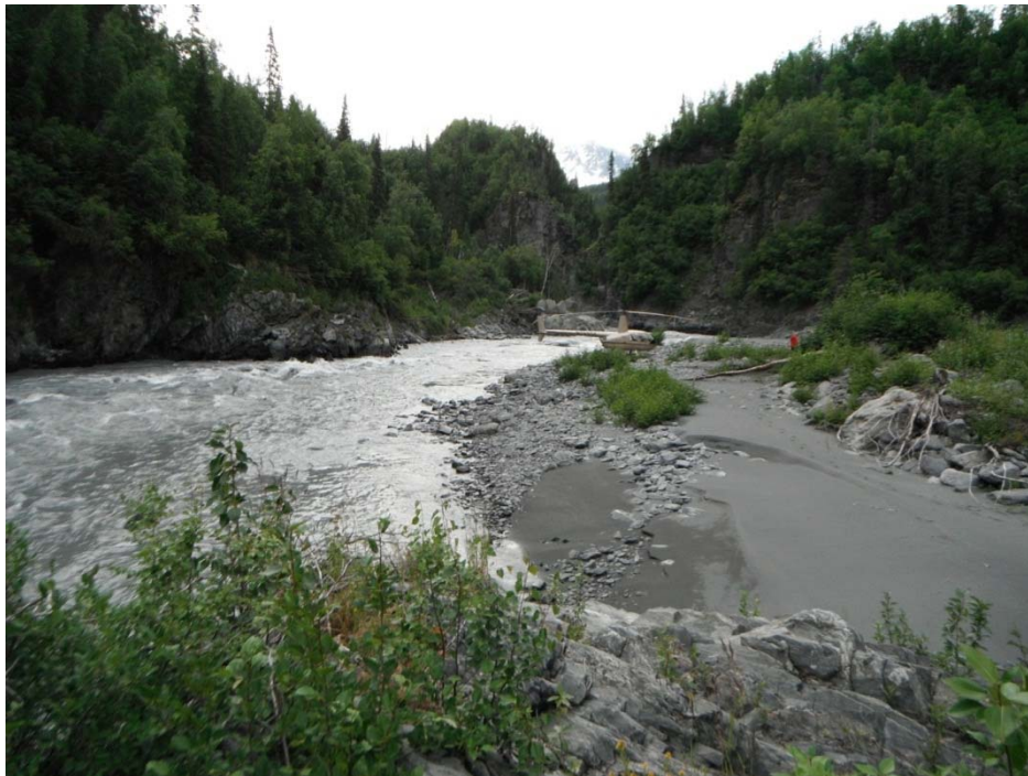
Figure 4-8 Scenario 1B, 3A Powerhouse – View Downstream (Photo 7-30-12)
